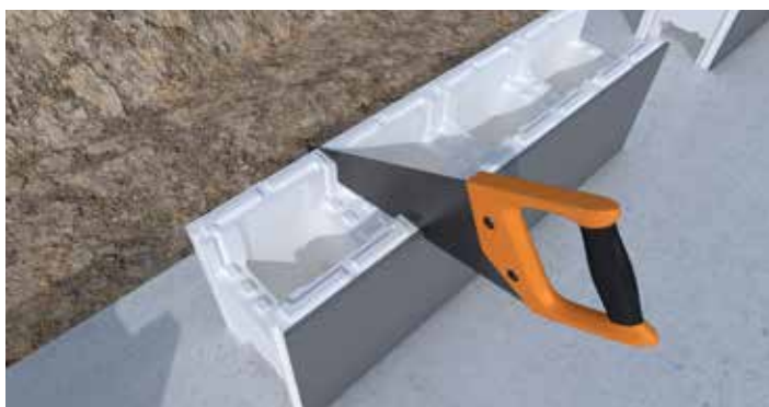
11 If you have to make a cut in a block, always cut in the middle of a spacer by following the markings
