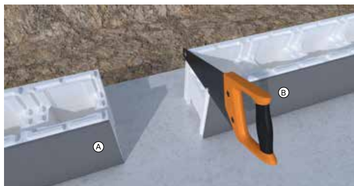
12 To assemble a recut block A, you have to cut the tenon of the block to be assembled B
