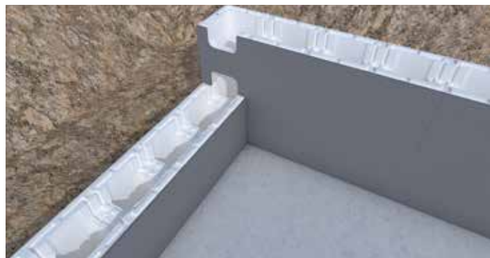
14 Assembly of the corner blocks of row 2
