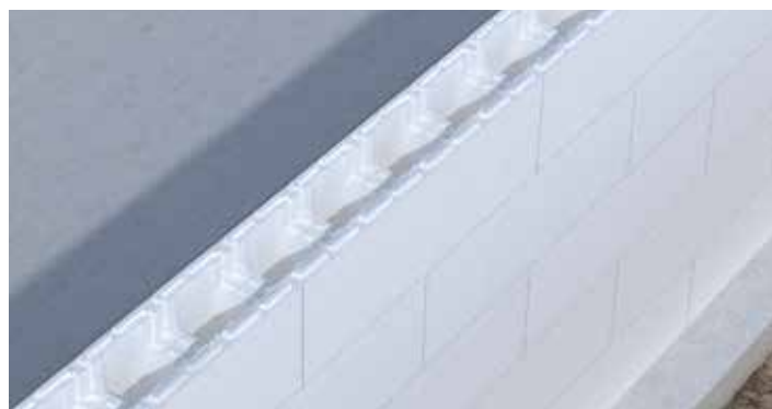
16 Wall of the assembled swimming pool. It is essential to cross the lower and upper elements by at least 25 cm
